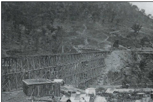
ABOVE: Running Water Creek - Company I constructed 4 blockhouses at this important Nashville and Chattanooga bridge in the Spring of 1864. Dunsmore might have reached his company in time to be among those working on the site. (Miller, Photographic History)
