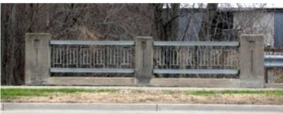
This is the most genuine of the bridges, although both sides are corroded. Note: The decoration on the stanchions matches that on the Maple Street bridge. In addition, The original cable and stanchions survive.
