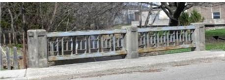
This bridge is quite corroded, especially the railing on the east side. The side cable supports are missing. Note: The decoration on the stanchions matches that on the Sixth Street bridge
